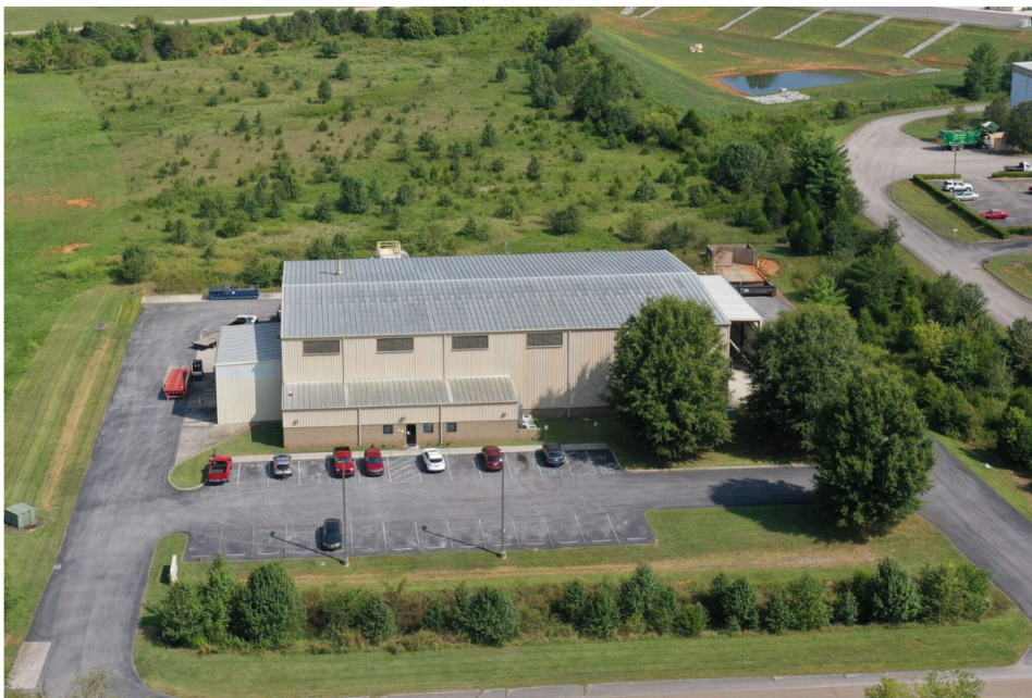
TreisD building. Courtesy of Mollenhour Gross Real Estate
